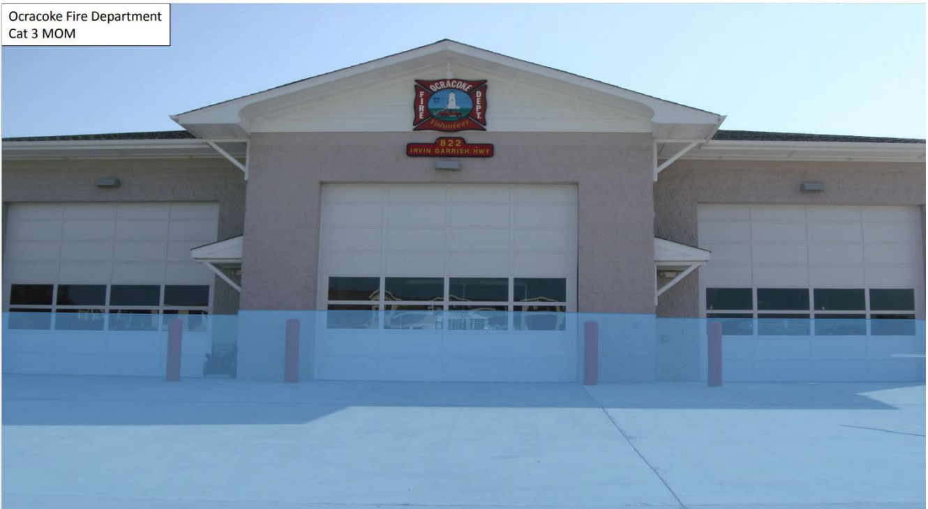
Figure 12: Category 3 Maximum of Maximum Storm Surge Inundation (Water Height Represented by Pale Blue Line) at the Ocracoke Fire Department, Ocracoke Island (FEMA 2016)
