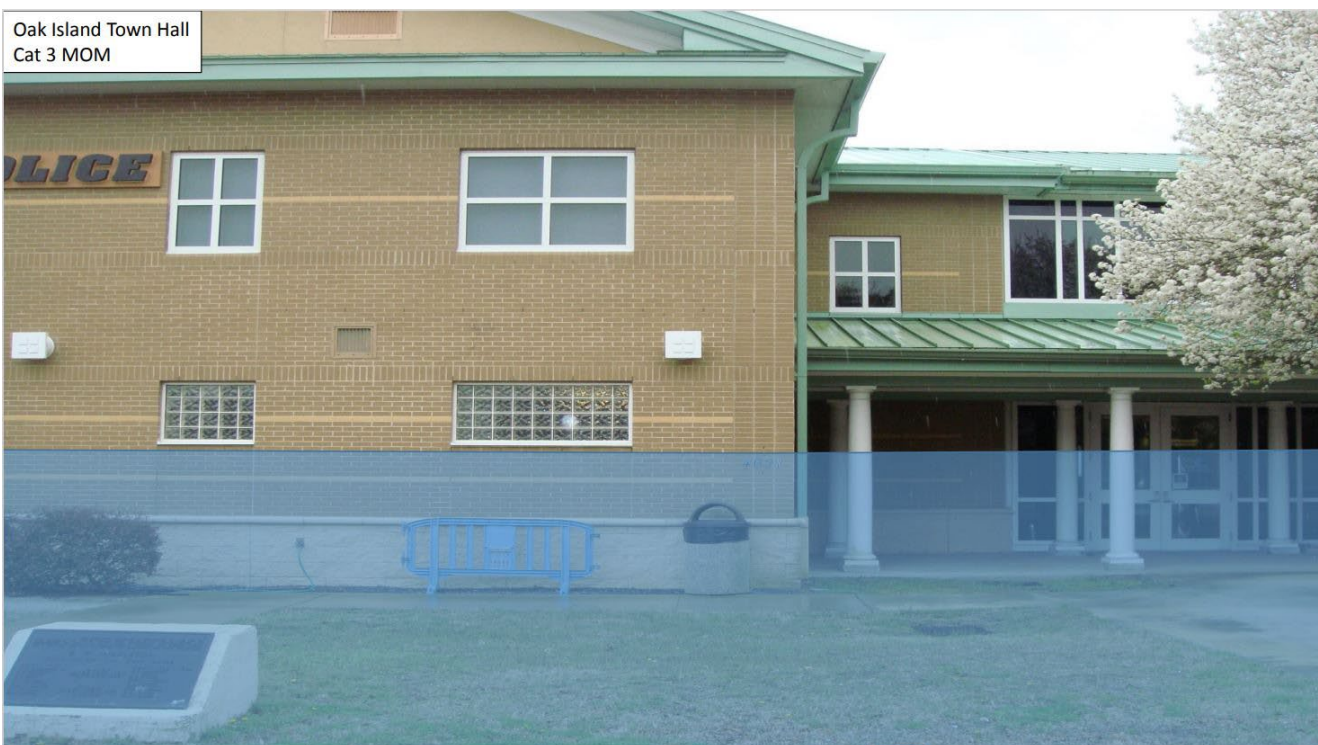
Figure 17: Category 3 Maximum of Maximum Storm Surge Inundation (Water Height Represented by Pale Blue Line) at the Town Hall in Oak Island, Brunswick County (FEMA 2016)
