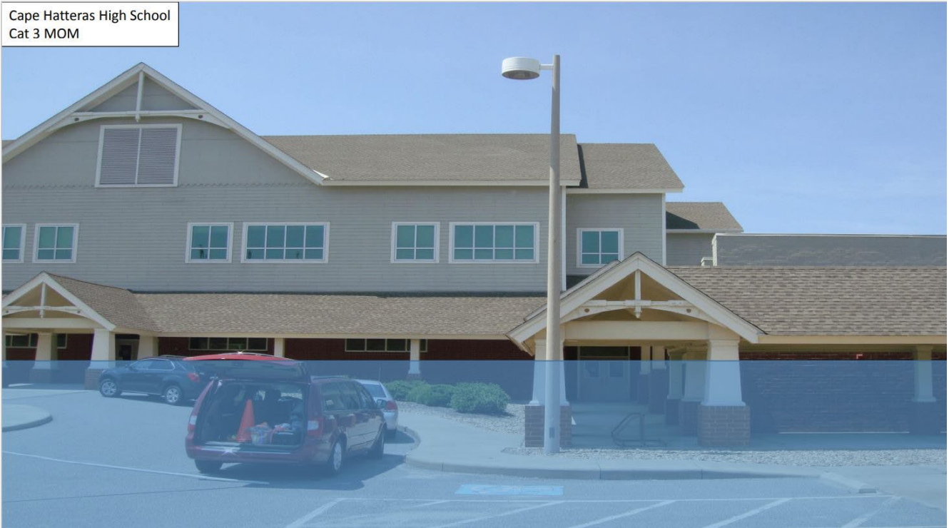
Figure 11: Category 3 Maximum of Maximum Storm Surge Inundation (Water Height Represented by Pale Blue Line) at Cape Hatteras High School, Dare County (FEMA 2016)
