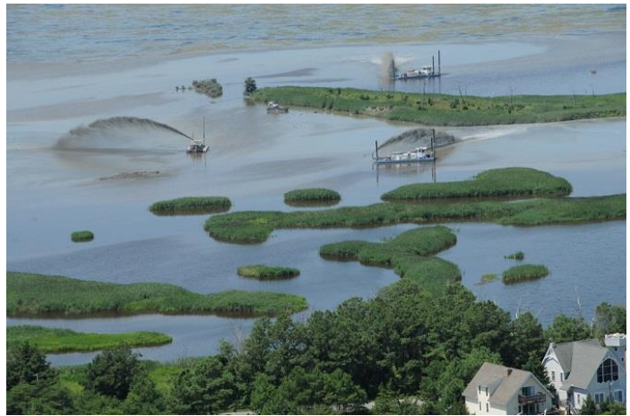
Figure 5-22: Thin Layer Placement (Photo Source: USACE ERDC)
