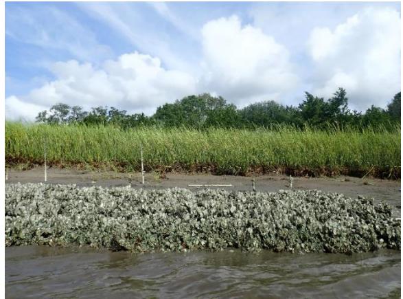
Figure 6-15: South Carolina Oyster Shell Living Shoreline Reef (Photo Source: South Carolina Department of Natural Resources)
