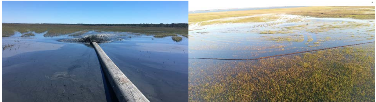
Figure 57. Construction of TLP site for AIWW project at Jekyll Creek, GA illustrating placement with an open 18" pipe (left) and distribution of sediment across the five acre site contained with coconut coir logs (right).
